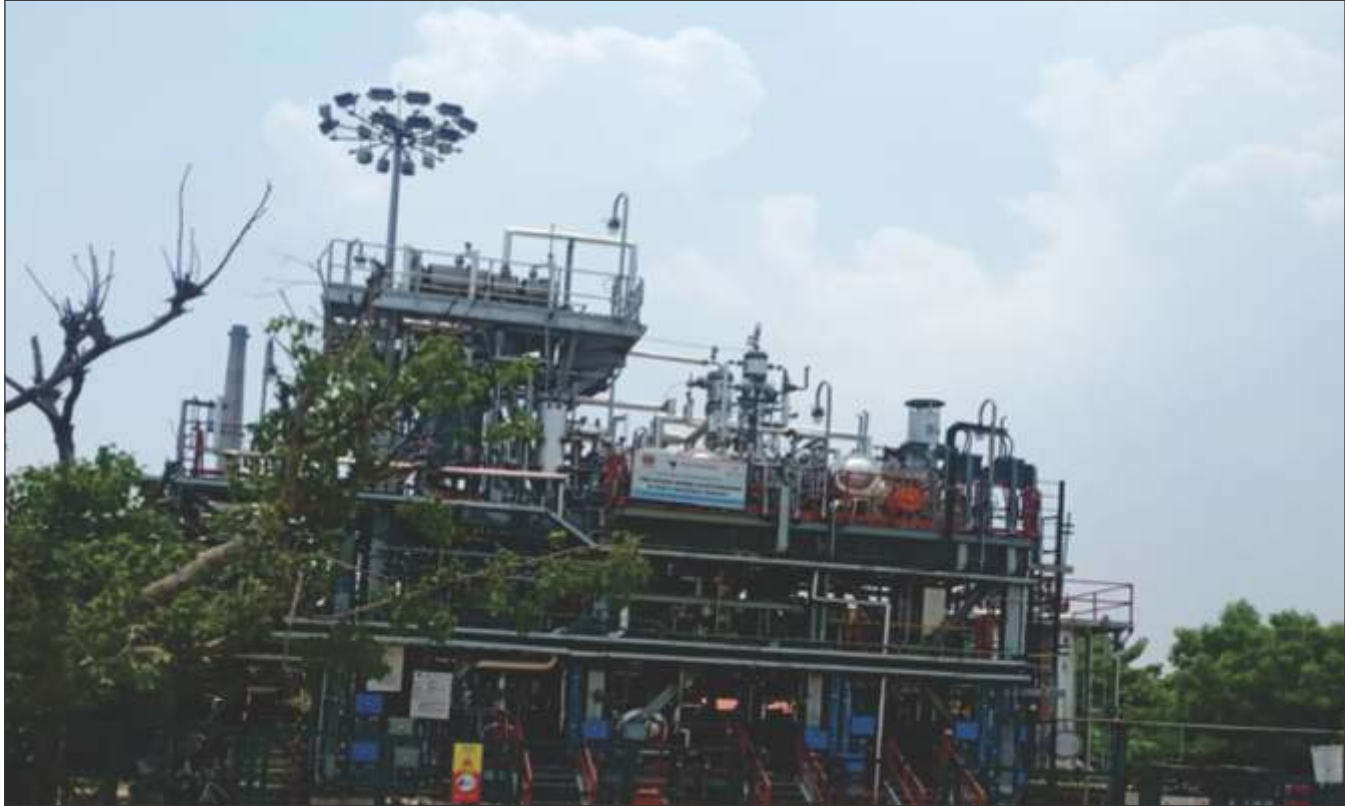
H-CNG Plant, IOCL
