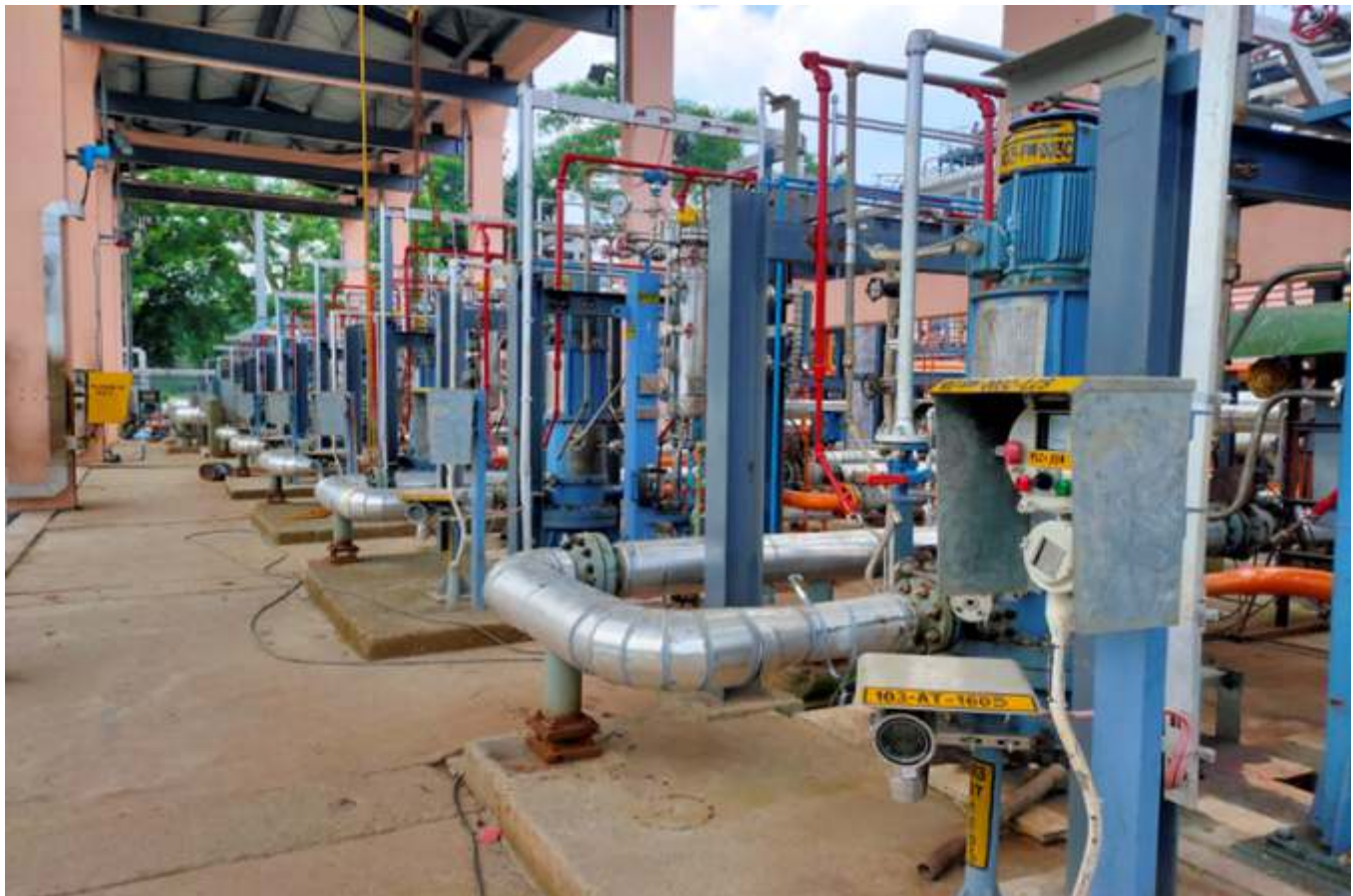
Utilities & Offsite - INDMAX Project of OICL
