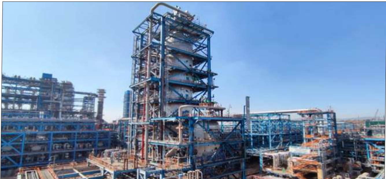
FCHCU STAGE-I & STAGE-II REACTORS
