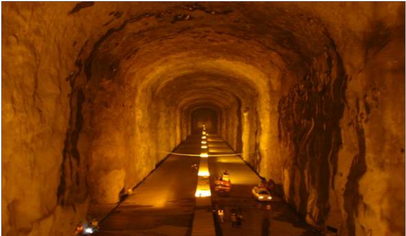
Cavern at Padur during construction
